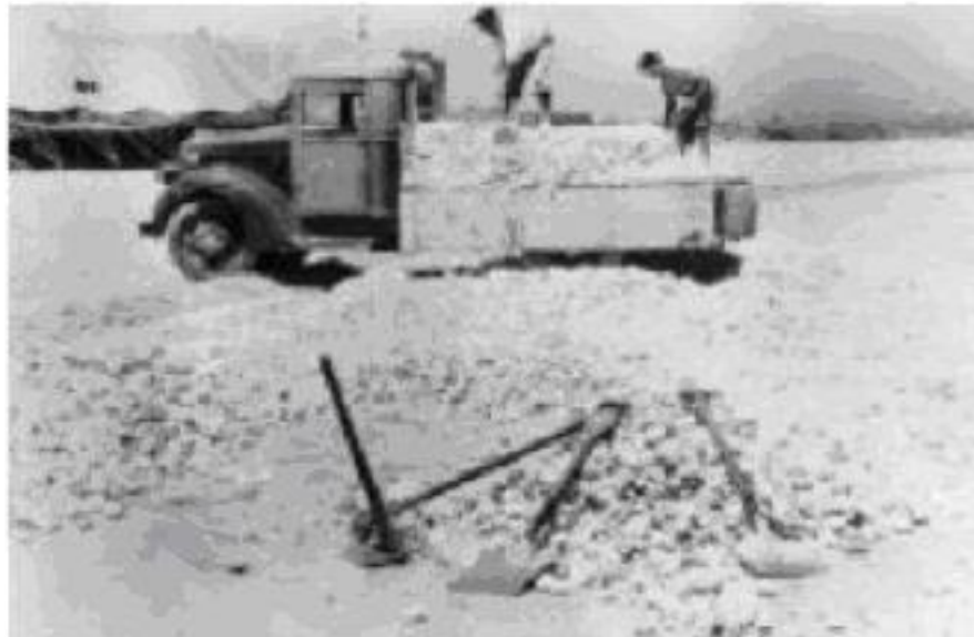
Maltese civilians repair airfield August 1942
